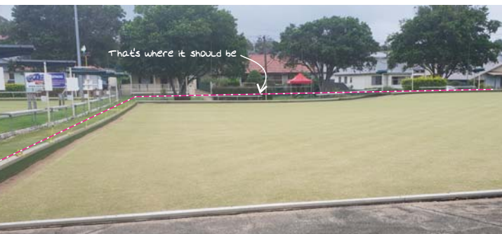
Above: Wallsend Diggers Sports Bowling Club Green collapsed from mine subsidence.
